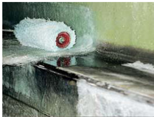
On the left Surface filler for levelling uneven surface.
